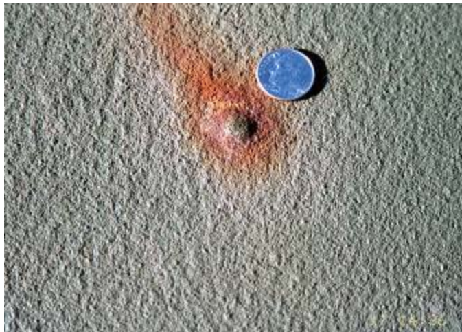
Figure 2 - HMA Failure: Pyrite eruption through acrylic coated HMA
